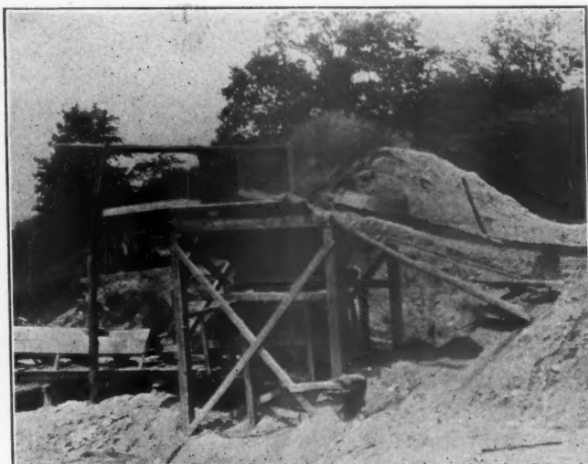
Receiving Hopper with Scraper Ready to Discharge
